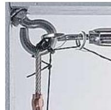
Corner fixings should also be attached with netting corner ties for extra strength.
